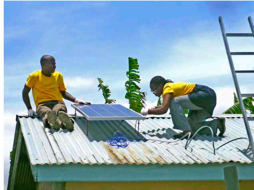
Installation of a solar home system in Tanzania
