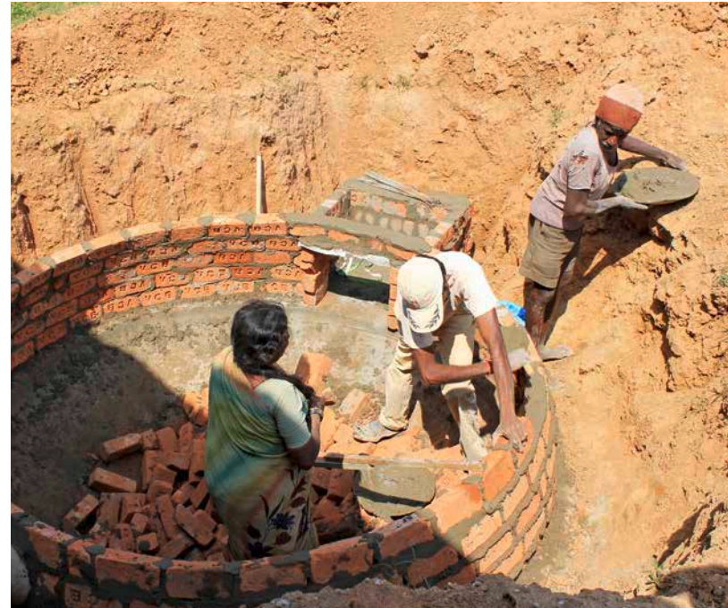
Construction of a biogas plant in rural India
